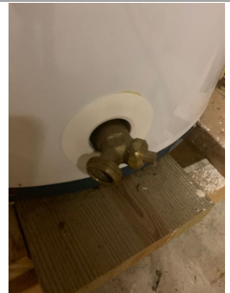
No handle for operating the discharge valve. Recommend plumber repair.
