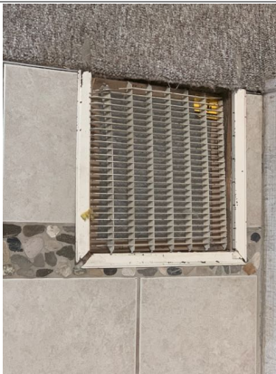
Cracked register on the southern side of the living room.
