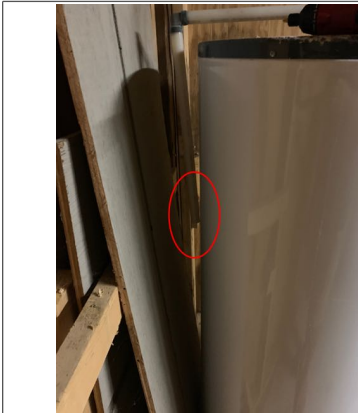
Temperature pressure relief valve doesn't terminate within 4" of the ground. Recommend plumber repair.
