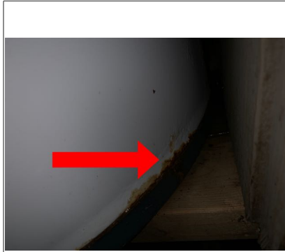
Rusting at the base of the water heater. Have plumber re-evaluate before closing agreement.
