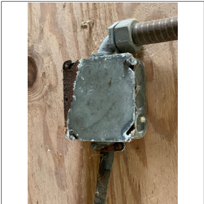
Rusted junction box at underside of carport ceiling, recommend licensed electrician replace.
