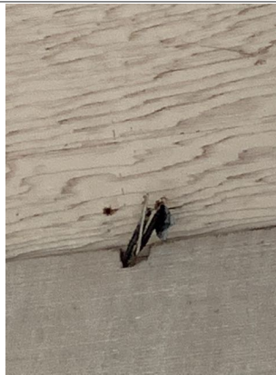
Exposed wiring at the southern wall above the main door. Recommend licensed electrician repair.
